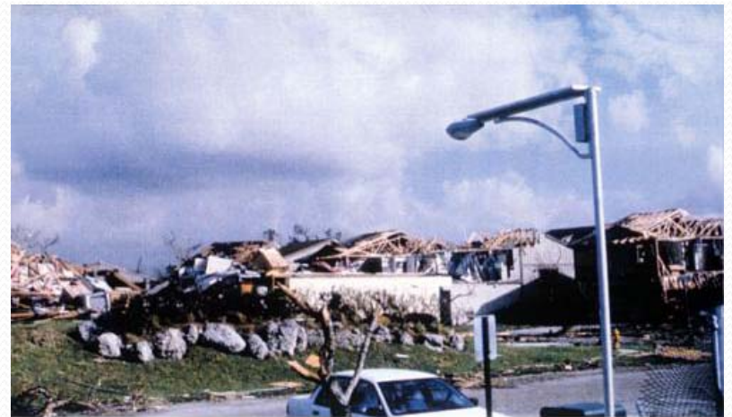
After Hurricane Andrew, Picture facing N.W.
